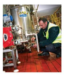
pump from Watson-Marlow Pumps. "The peristaltic operating principle intrigued us, because it seemed there would be no way to introduce oxygen into our process," comments Evans. "However, the proof is in the pudding, so we introduced an SPX25 model to one of our filter mains."
